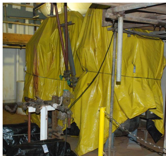
Water treatment cover with canvas – FRADE HULL
